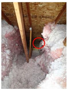
**Repair:** Openings into the attic space from the roof surface are evident where the west living room roof intersects the ridge of the east facing roof (under the overhang along gable wall) at both sides. The openings allow entry for bird or rodent intrusion into the attic. Recommend blocking the openings with wire mesh or other material to prevent any intrusions.
