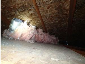
**WDO:** The three bathroom ceiling exhaust fans leak air into the attic space because incorrect roof vent type is lacking a collar to secure the vent connection resulting in moisture stained sheathing that is testing at elevated moisture levels. Recommend replacement of existing non collared box vents with collared roof vent followed by positive connection of ducting to eliminate damp air venting into the attic space.
